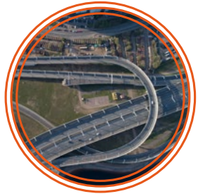
Construction of a section of Makarov embankment with exits from the Western High-Speed Diameter to Vasilyevsky Island
