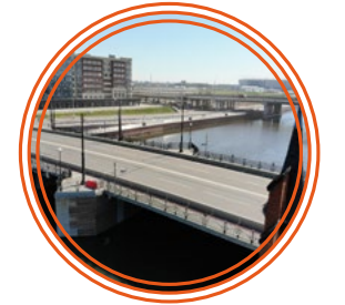
Reconstruction of the Vysoky drawbridge in Kaliningrad, as well as the construction of Veteranov embankment and a pedestrian tunnel
