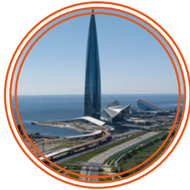
Construction of streets bordering the Lakhta Center quarter and adjoining Primorskoye Chaussee, as well as construction of overpasses
