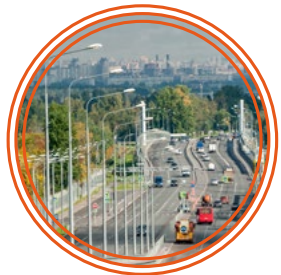
Construction of a road bypass in Krasnoye Selo
