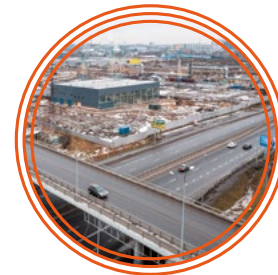
Construction of an interchange with Murmansk highway in Kudrovo
